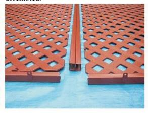
Slide on the top C-Channels and fit plastic moulded corner in each end. Then slide the H-joiner up between the two sheets to be joined.
