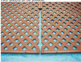
Gently tap the plastic corners into the H-Joiner to secure the sheets together.
